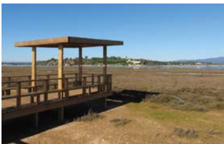
Wood structure (footbridges and rest area) on the route "Ao Sabor da Maré".
